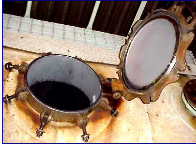
CYCLETIGHT® RCM-Type 6 (Secures to Manway Nozzle)
